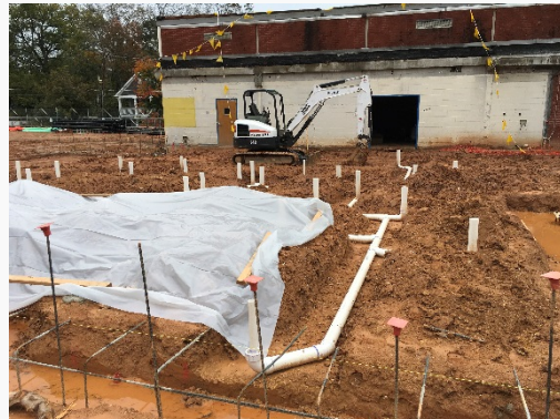
Underground Plumbing Rough
