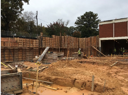
Complete Retaining Wall Formwork
