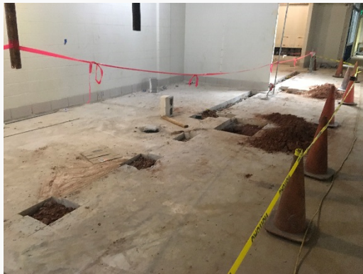
Sawcut Slabs to Install Plumbing
