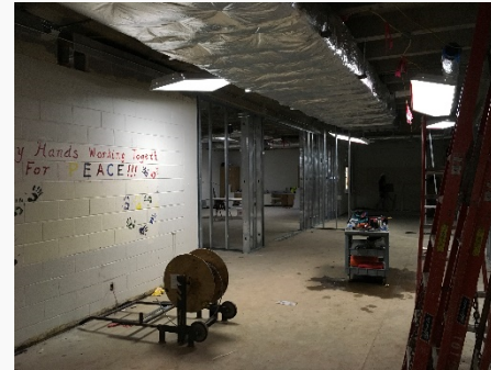
Interior renovation MEP rough and framing / drywall
